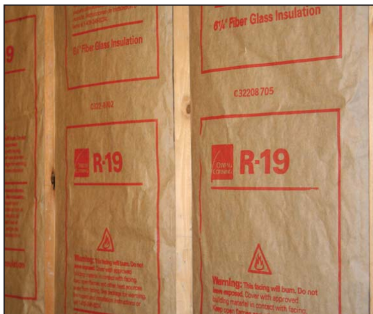
Properly installed inset-stapled fiberglass insulation, resulting in a Grade I rating.
